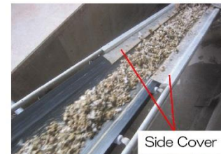
Preventing scattering of manure at the edge part of the belt
